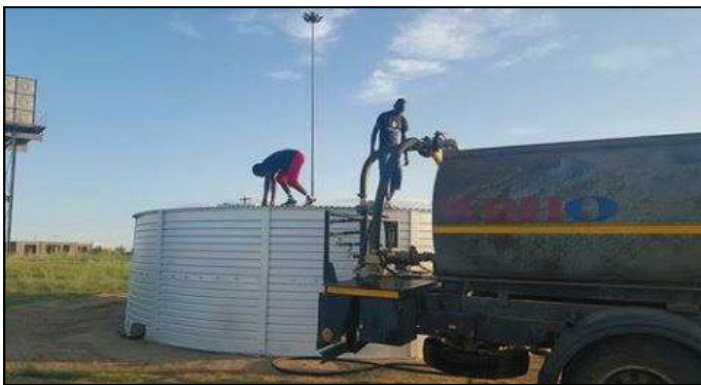
Workers filling up the tank with water from Reitz
